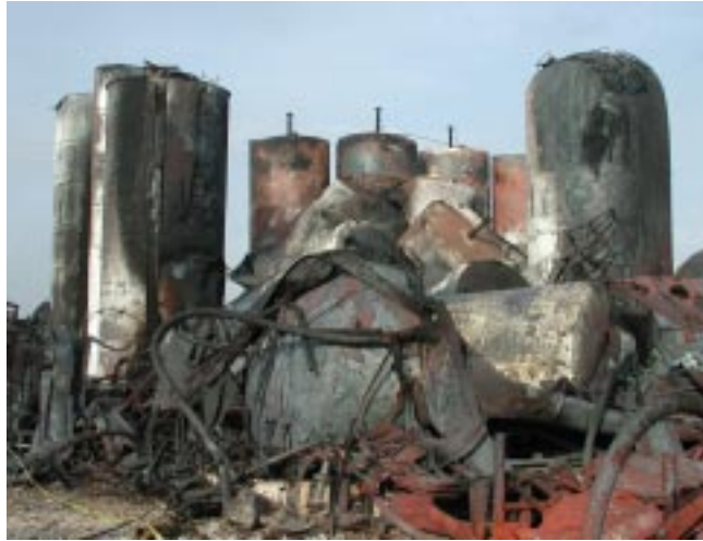
Figure 9. Failed storage tanks.
