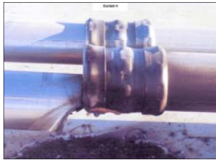
Fire at Mercantile Occupancy, California, April 2009
