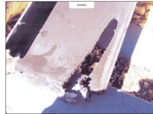
Fire at Mercantile Occupancy, California, April 2009
